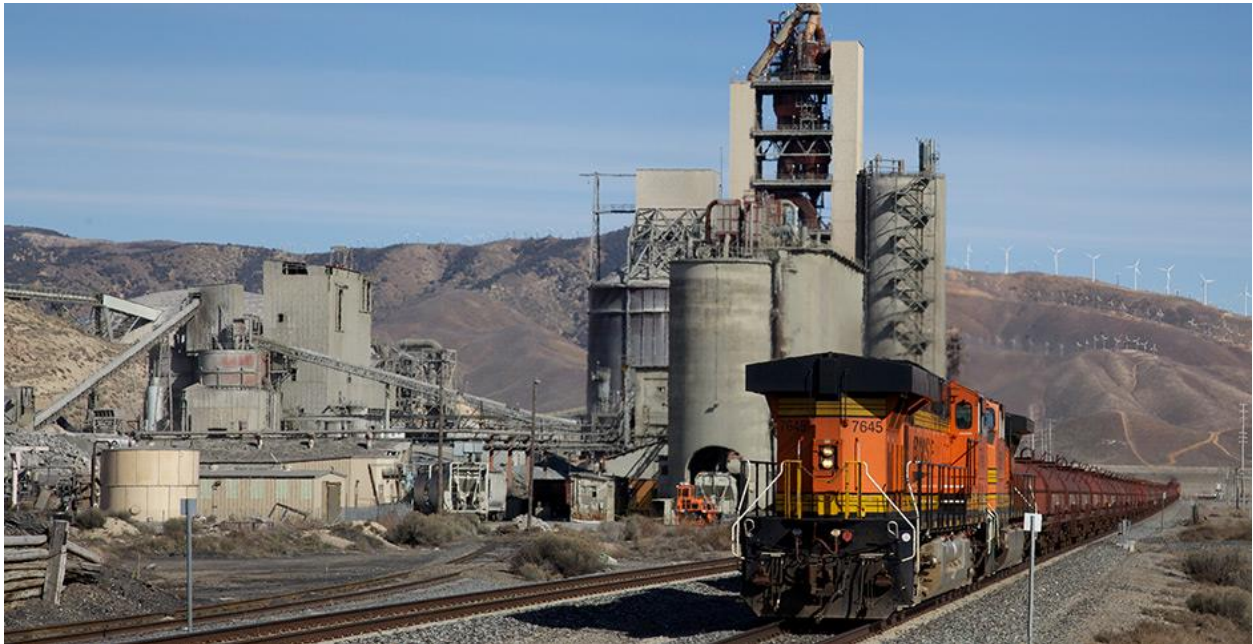
The Lehigh Southwest Cement plant in Tehachapi, Calif., burns coal to cook limestone mined from nearby hillsides. Photo credit: David Brossard/Flickr
